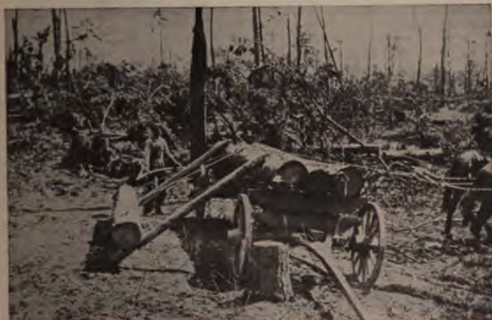
FIG. 50. — Loading a Log Wagon by means of the Cross-haul. Missouri.
